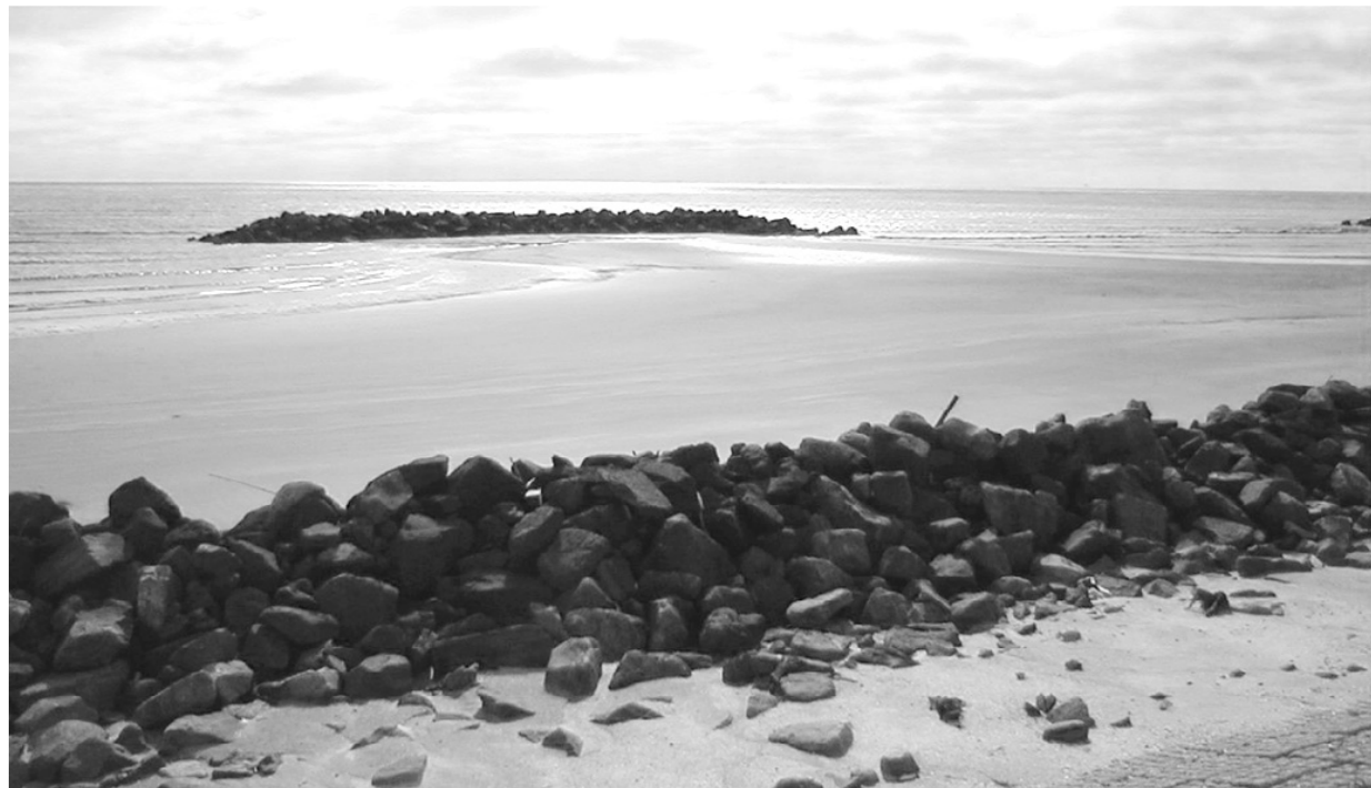
A STRONG NORTH wind last week combined with a low tide had the area between the shoreline and the breakwaters almost high and dry west of Holly Beach. The breakwaters were built to try to stop the erosion of beach between Holly and Constance beaches and to help rebuild the beaches. Some improvements along this line have been noted.
