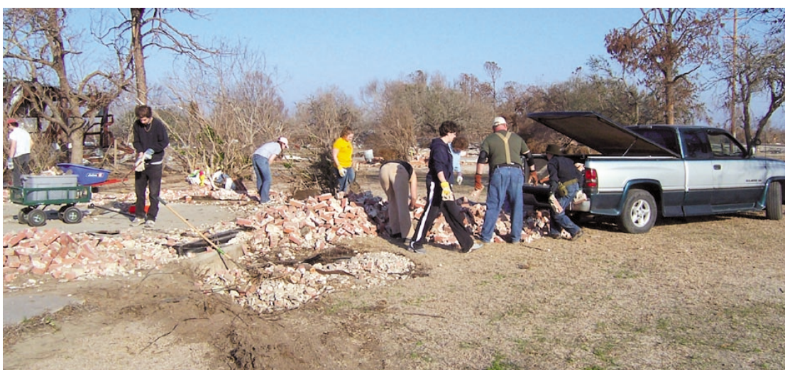
STUDENTS FROM Anna Maria College in Paxton, Mass., are in Cameron helping residents clean up. On Tuesday they were at Chris Mooney's home moving bricks. The college has two other Habitat for Humanity groups working this week, one in Miami, Fla., and the other in Austin, Tex. (Photo by Cyndi Sellers.)
