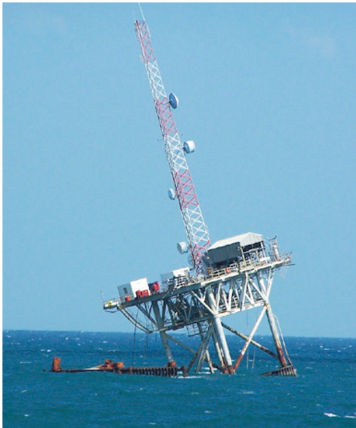
IN ADDITION to the devastation left in Cameron Parish, Hurricane Rita caused great damage to oil rigs located off the Cameron coast. Above is one such rig which is still standing, although greatly bent. (Photo by Capt. Sammie Faulk.)
