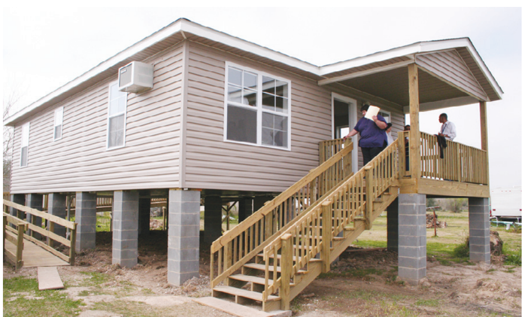
THE HOME OF Mitchell and Carolyn Hebert of Hackberry was dedicated Thursday, March 6 by Mennonite Disaster Services. It is the second MDS home to be dedicated in Cameron Parish this year, with two more to follow. (Photo by Cyndi Sellers.)
