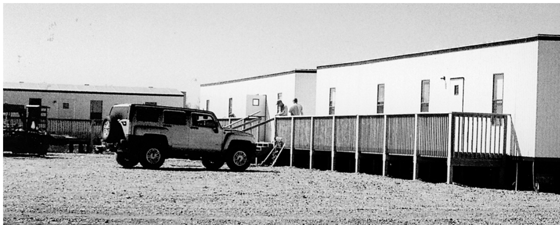
THE CAMERON PARISH Police Jury's temporary office in Grand Lake, shown being readied for occupancy, is located just south of the Parish line on the Gulf Highway in Grand Lake. (Photo by Cyndi Sellers.)
