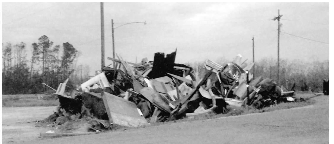
ABOVE IS THE remains of DeBarge's Convenience Store in Hackberry following Hurricane Rita. John DeBarge, who had the store over 23 years, said he does not plan to rebuild.
