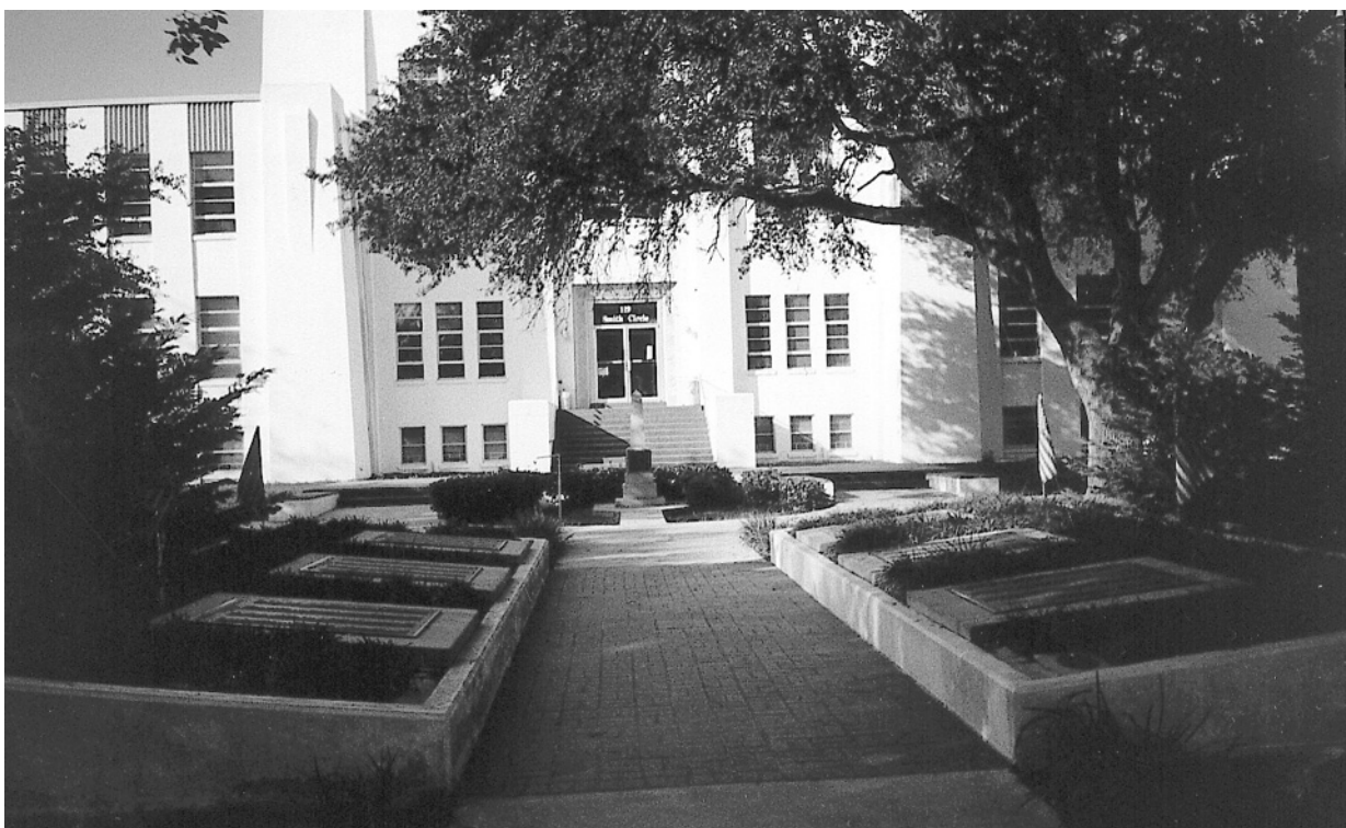
THE CAMERON PARISH Courthouse is 64 years old and still is in full use by parish offices (although some have had to move into other buildings due to a need for more space.) It was one of 12 new courthouses built in Louisiana from 1937 to 1940 as WPA projects. The plaques in the foreground list Cameron Parish residents who served during war time and in front of the courthouse is a monument to the parish's war dead.
