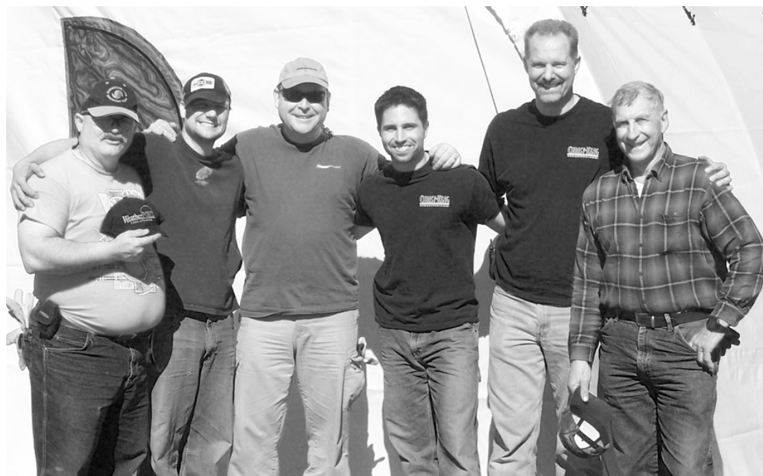
A TEAM OF volunteers from Lynden, Wash., was in Cameron last Friday to install a tent for the First Baptist Church. Local church members Paul Sellers, left, and Charles Primeaux, right, are pictured with volunteers Cliff Tadema, Gerrit Boyle, Lance Ellis, and Sean Taylor. (Photo by Cyndi Sellers.)
