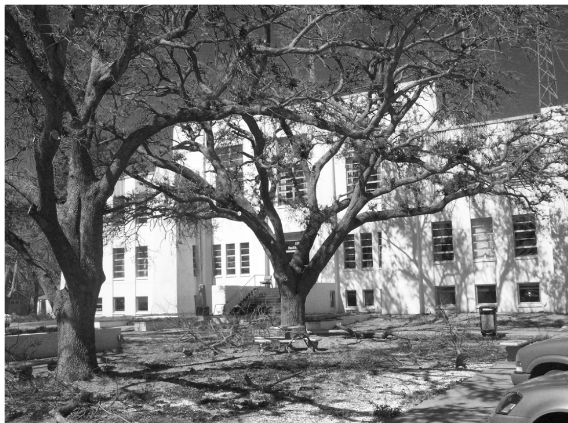
ALTHOUGH THE town of Cameron was almost wiped out by Hurricane Rita six months ago, the Cameron Parish Courthouse was relatively undamaged except for the lower floor/basement which was flooded. The courthouse, which was built in 1937, also survived Hurricane Audrey in 1957, also without much damage.
