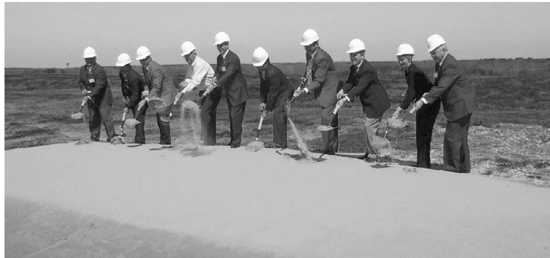
FEDERAL, STATE and local officials joined officers of Cheniere LNG, Inc. to break ground for the company's Sabine Pass LNG Terminal, March 23rd in Johnson Bayou. Taking part were: Cheniere LNG President Keith Meyer, Cheniere Energy CEO Charif Souki, Louisiana Dept. Of Natural Resources Secretary Scott Angelle, Louisiana Dept. of Economic Development Secretary Michael Olivier, FERC Chairman Pat Wood, FERC Commissioner Suedeem Kelly, U.S. Rep. Charles Boustany, State Sen. Jerry Theunissen, Cameron Parish Police Jury President Scott Trahan, and Johnson Bayou/Holly Beach Juror Sonny McGee. (Photo by Cyndi Sellers.)
