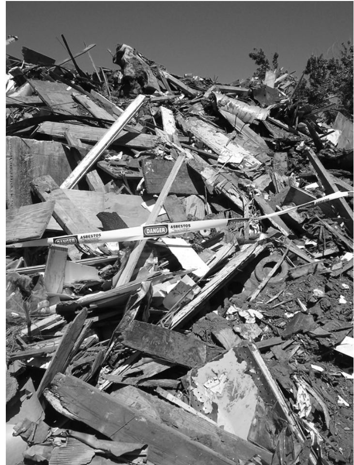
THIS PRIVATELY demolished building contained asbestos and was tagged for special treatment. OSHA requirements for worker safety outline a process for asbestos removal that includes wetting the pile, wearing protective equipment, hand separation, double-bagging, and removal of asbestos to a Type I or II disposal site. (Photo by Cyndi Sellers.)
