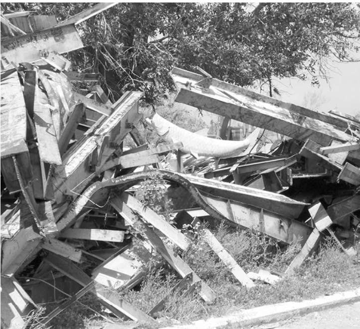
THE SOUTH CAMERON Tarpon statue can be seen in the midst of the piles of steel coming from the demolition of the school. (Photo by Cyndi Sellers.)
