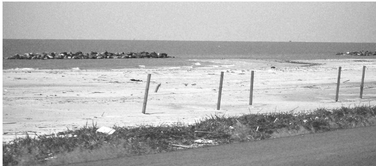
RESTORATION OF the sand dunes, which once covered the fences on the beach, is set to begin with plantings of beach grasses. Funding for replacing the lost sand is being sought. The combination of breakwaters and beach nourishment has been considered a success, as Hwy. 82 did not wash away during Hurricane Rita. (Photo by Cyndi Sellers.)
