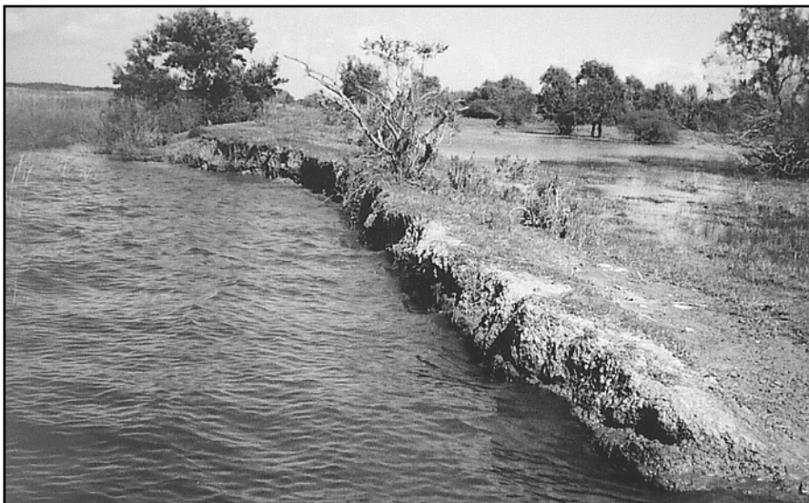
Levees along Mermentau River and adjacent property Outer Protection Levees
