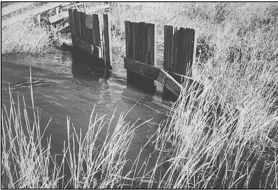
Water Control Structures along the Mermentau River at Upper Mud Lake
