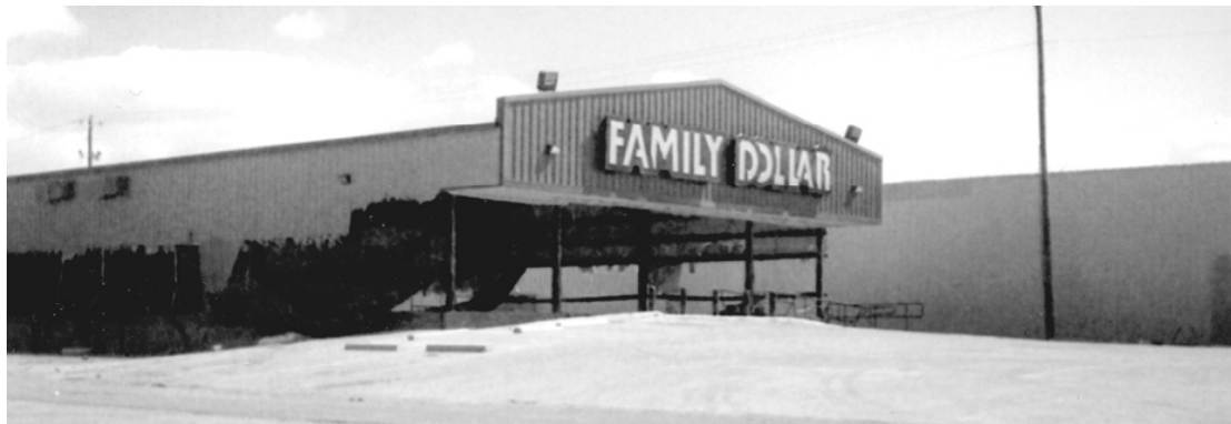
THE FAMILY DOLLAR Store in Cameron was completely gutted by the water and winds of Hurricane Rita. (Photo by Grace Welch.)
