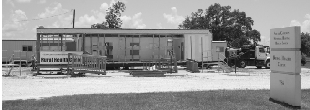
DISASSEMBLE. . . REASSEMBLE. The South Cameron Memorial Hospital Rural Health Clinic at Grand Lake is being moved to a rent-free parish owned site on Eighty Acres Lane. The four sections of the modular building, placed in Grand Lake after Hurricane Rita to accommodate displaced patients, were being separated on Saturday and moved to the new site. It is expected to be in operation again in the near future. (Photo by Cyndi Sellers.)
