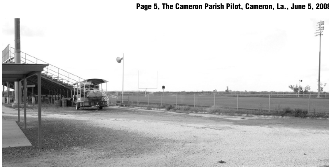
THIS SMALL AREA at South Cameron High School will hold two restrooms and a concession stand, following the granting of an elevation variance by the Cameron Parish Police Jury Monday night. The foreground is a driveway which cannot be used for the buildings.
