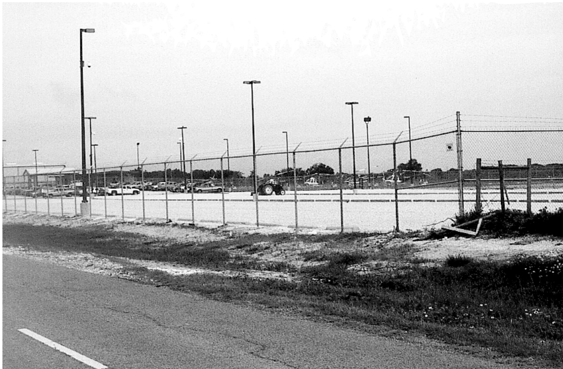
AIR LOGISTICS is expanding its Cameron helicopter facilities on Trosclair Road. The expansion covers six acres with eight new helipads and 250 new parking spaces. The expansion is due to increased demand for the company's helicopter services in the oil and gas area. (Photo by Cyndi Sellers.)
