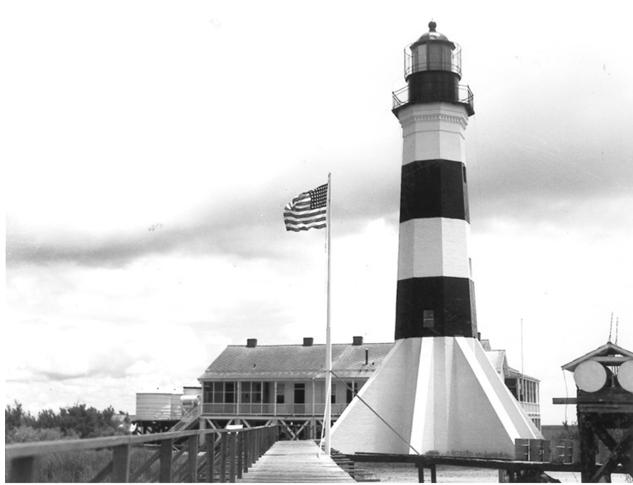
THE SABINE PASS LIGHTHOUSE is pictured above as it looked in years ago before the keeper's house burned in a grass fire and vandals stole the copper roof. The lighthouse now has new owners, the Cameron Preservation Alliance, which hopes to restore it and possibly establish a state or national park at the site.
