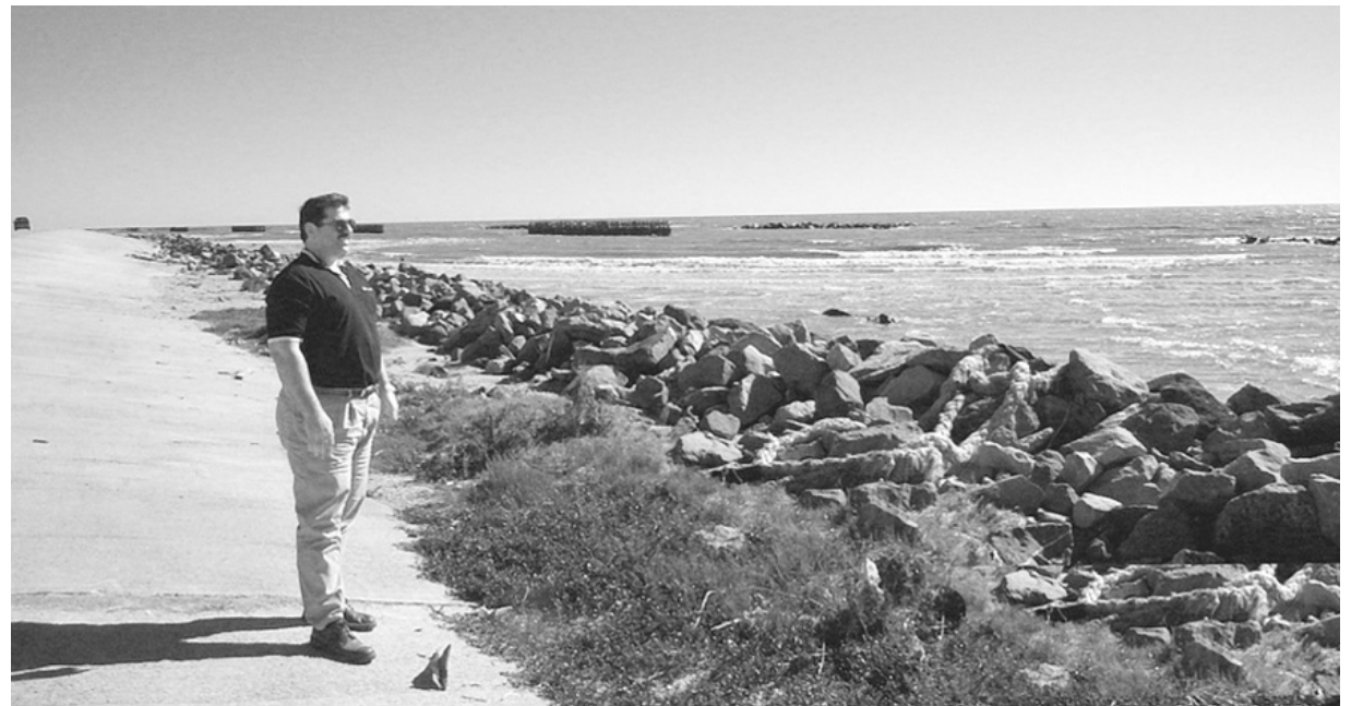
A VISITOR, Allen Danos of Galliano, here views the rock breakwaters between Holly Beach and Constance Beach which were recently built higher as part of a beach restoration project. In a few weeks a contractor will begin pumping sand from offshore between the barriers and the beach which, it is hoped, will stabilize the beach and provide additional protection to the highway and to the beach homes in the area.
