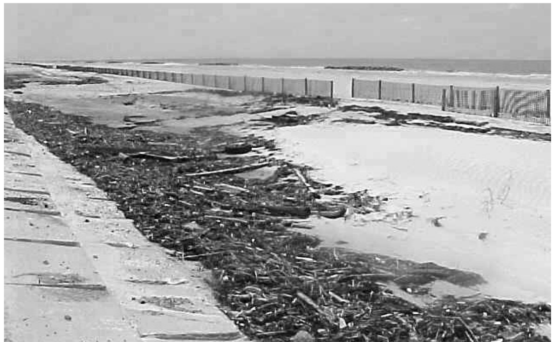
THIS PICTURE shows the debris that was washed up on the beach by Hurricane Claudette recently. However, the sand fence in the background prevented a major loss of the new sand that has been put on between Holly Beach and Constance Beach this past year. (Photo by Dede Nunez.)
