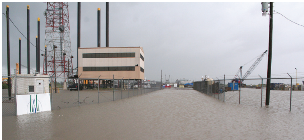
PARKING LOTS along the Cameron docks were under water for a time. (Photo by Cyndi Sellers.)
