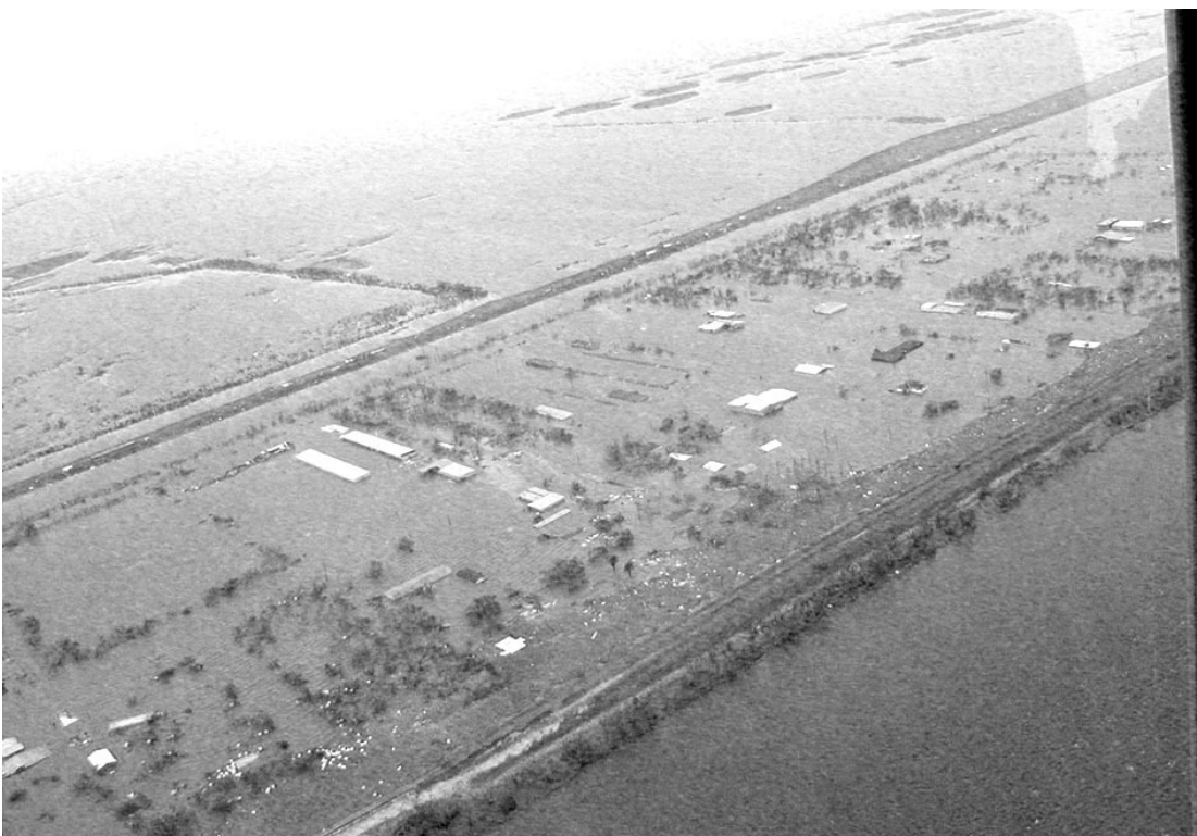
ERA HELICOPTERS, which has an operation in Cameron, suffered severe damages at its Venice facility from Hurricane Katrina, as the above photo shows. Eight of the ERA employees there lost their homes and a local collection is being made to aid the employees directly affected by the storm. Anyone wishing to make a donation may send it to the attention of Wendy Mann; c/o Era Helicopters LLC; P. O. Box 6550; Lake Charles, LA 70606. Call 337-478-6131, extension 215 if you have any questions. (Photo courtesy ERA and Dede Nunez.)
