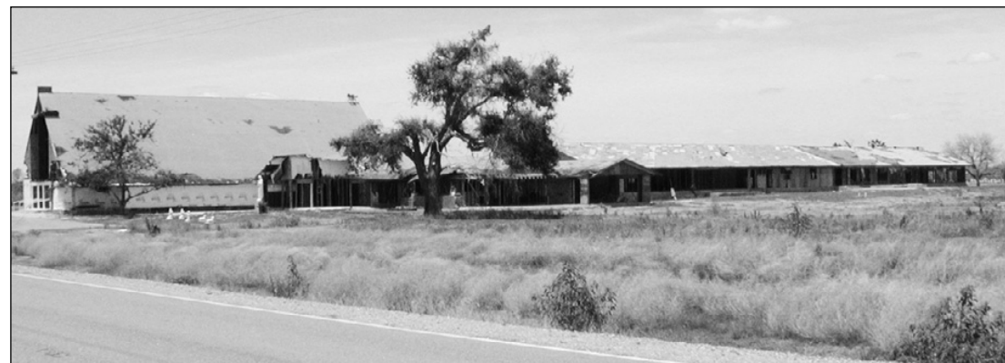
The entire physical plant of Sacred Heart was damaged. Here the church, rectory, hall and religious education building can be seen. The sides of the church were blown out by the surge of the water, which also devastated the rectory, hall and religious education building. Plans continue to be worked out on reconstruction of the church.
