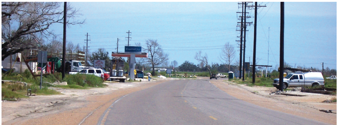
THIS IS CAMERON'S main street one year after Hurricane Rita. Rebuilding is underway. (Photo by Cyndi Sellers.)
