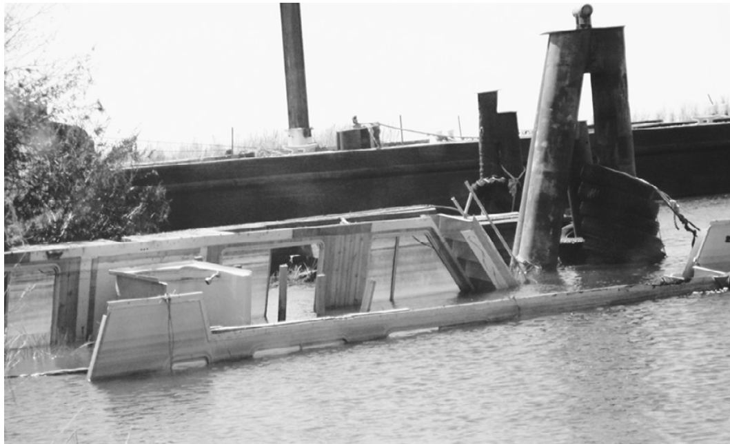
THIS HOUSEBOAT in Johnson Bayou sank because of Hurricane Ike.
