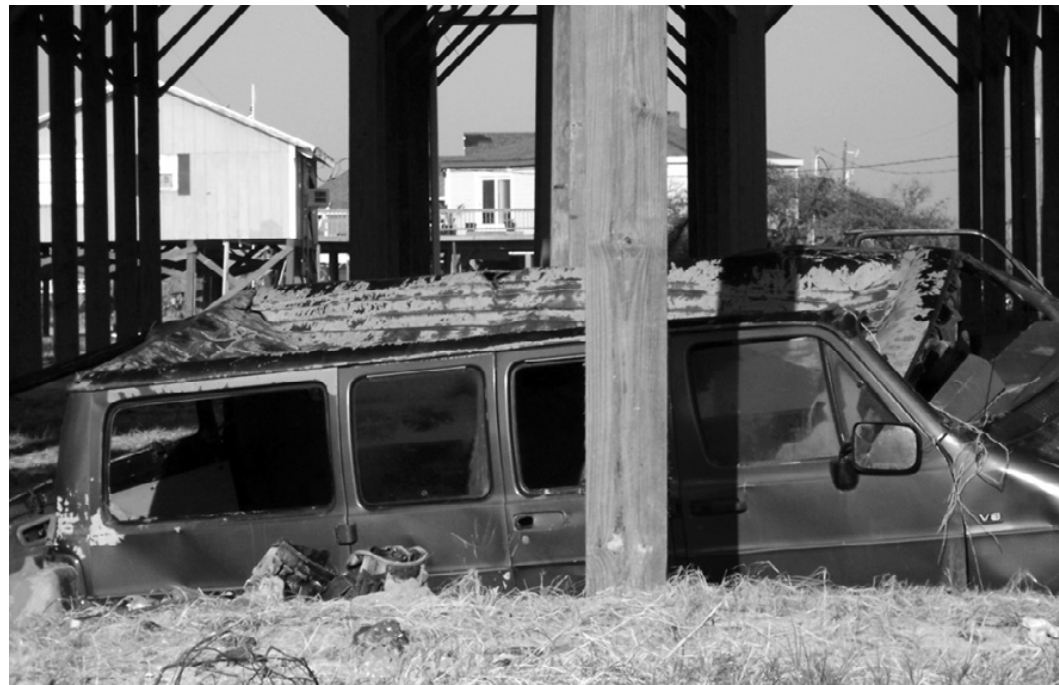
A VAN WAS buried in this scour hole left in Johnson Bayou by Hurricane Ike's passage through Cameron Parish.
