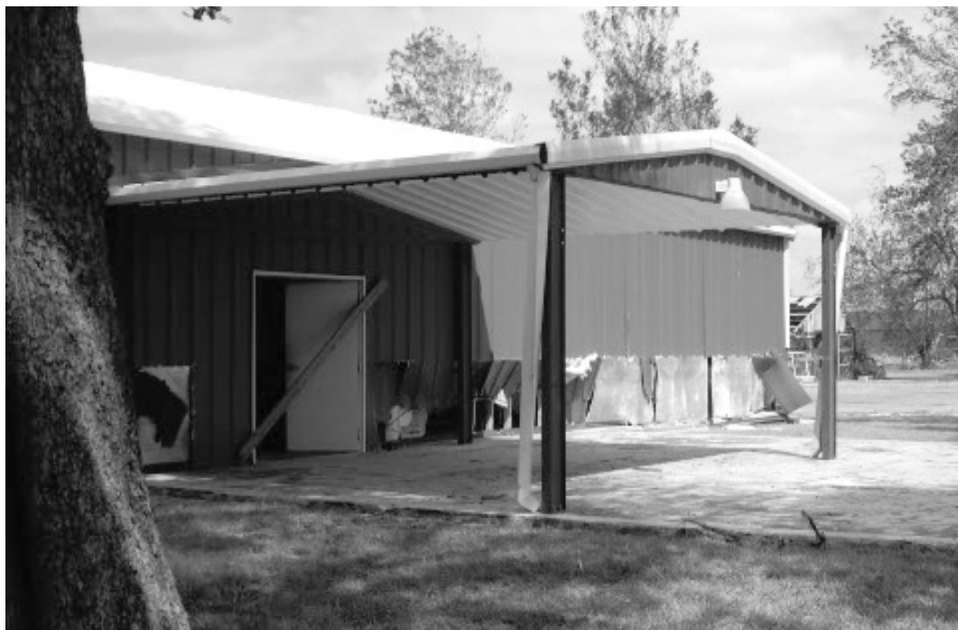
THE DAMAGES to the Oak Grove Baptist Church by Hurricane Ike are shown in the above photo. There was three feet of water in the church. The church parsonage was high and dry, as was the home of Wendell and Judy Rutherford who elevated eight feet after Rita.
