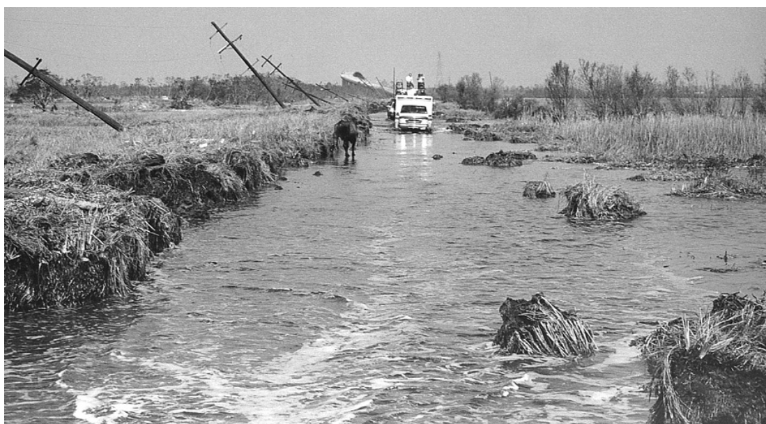
HWY. 27 south of the Gibbstown Bridge was covered with water on Monday, Sept. 26 as General Honore's convoy moved deeper into Cameron Parish to assess damage. Huge mats of marsh grass covering the roadway had to be cleared ahead of the vehicles. (Photo by Mike Sellers.)
