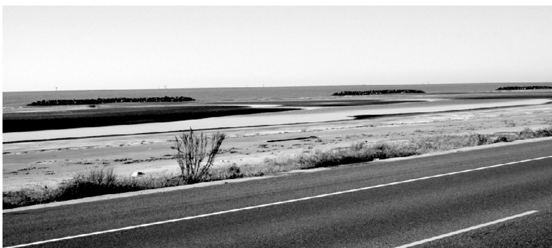
THE NEWEST breakwaters along LA 82 are working well, as seen in the low tide photo. More breakwaters are being considered as part of the coastal protection plan for Louisiana. (Photo by Cyndi Sellers.)
