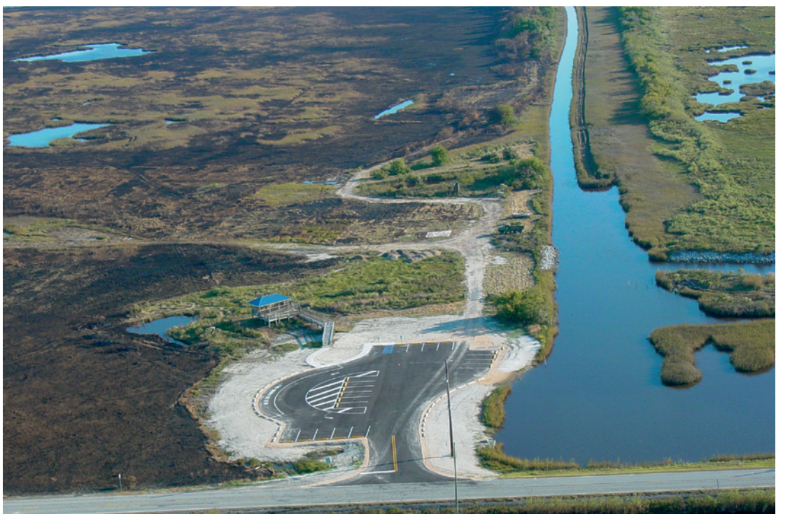
THIS AERIAL photo shows the new wildlife observation tower, parking area, and Blue Goose Trail which will be dedicated on Wednesday, Dec. 17 at the Sabine Wildlife Refuge south of Hackberry.
