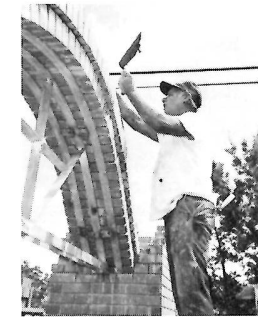
Robert Crador laying the bricks
