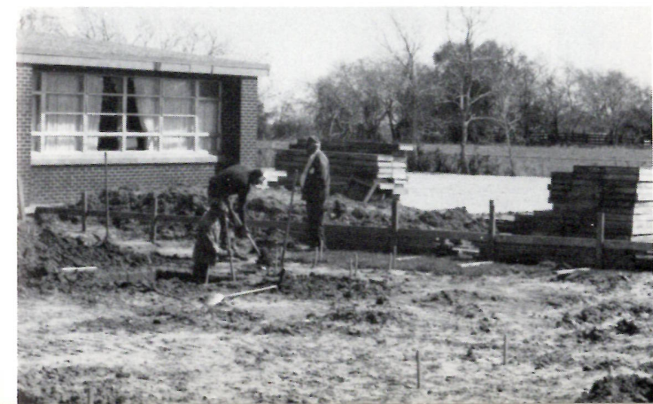
The construction workers install an underground pipe. The ground is being prepared for the pouring of cement.
